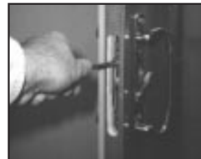
Adjusting the latch arm.
