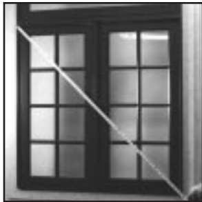
Making sure the frame is square.
