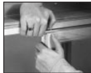
Removing the sash.
