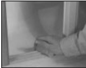
Lubricating the track with paraffin.
