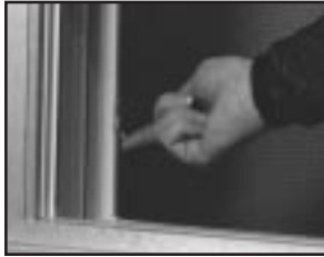
Lifting butterfly catch on screen.
