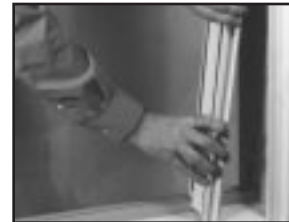
Slowly pull the bottom edge of jamb liner across sill and remove.
