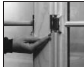
Lifting the sash lock lever.
