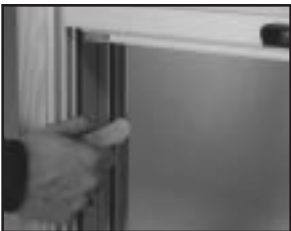
Lubricating the jamb liner with paraffin.
