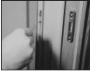
Adjusting the screen strike.
