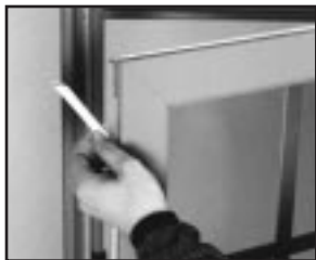
Removing the sash weather-strip.
