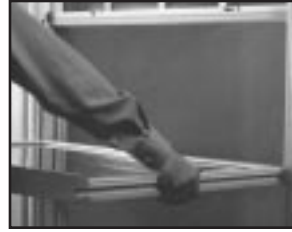
Removing the sash.
