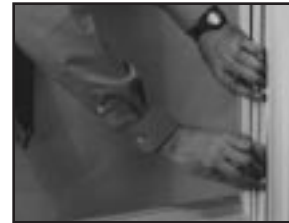
Compressing and disengaging jamb liner from frame.
